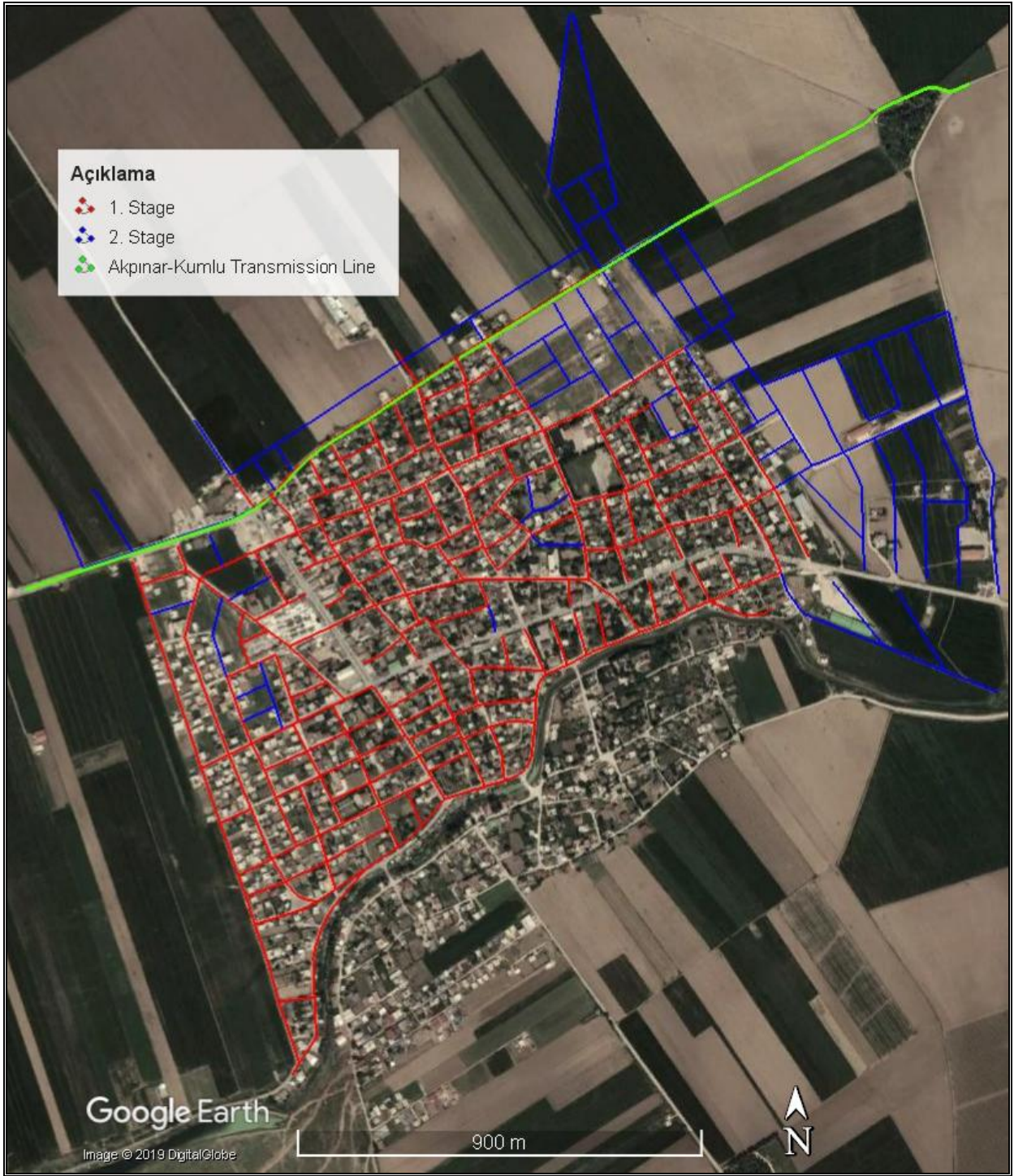
Figure 4: Kumlu Water Supply Network Pipes and Part of Transmission Line on Googleearth view
